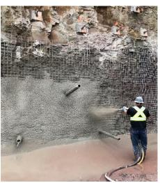
UNIQUENESS: WET MIX SHOTCRETE AND NEARLY 220 75MM DIA X 10M LONG ROCK ANCHORS POST TENTIONED USING A 100TON THROUGH HOLE JACK.
